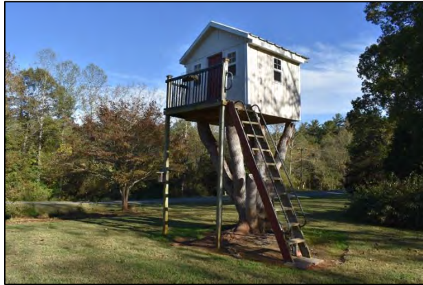
Figure 25: View of tree house looking to southwest.
