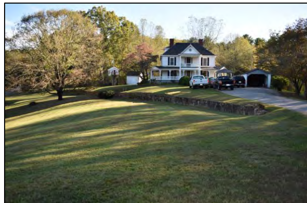
Figure 27: View of retaining wall, looking to south.
