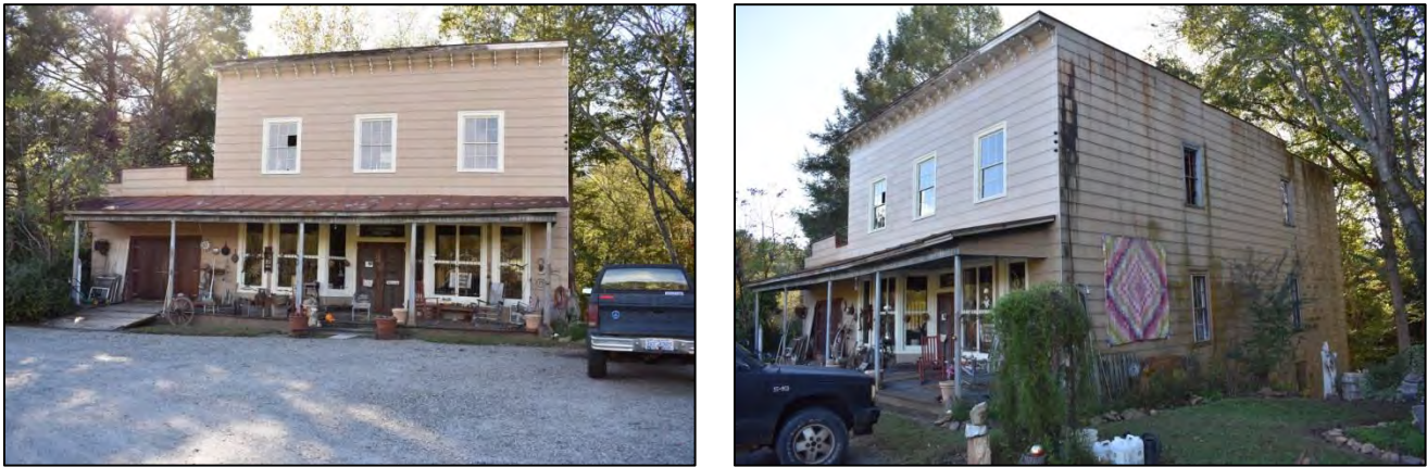
Figure 17: Left, front (eastern) elevation of Jennings Store; right, view of northeastern corner of store.
