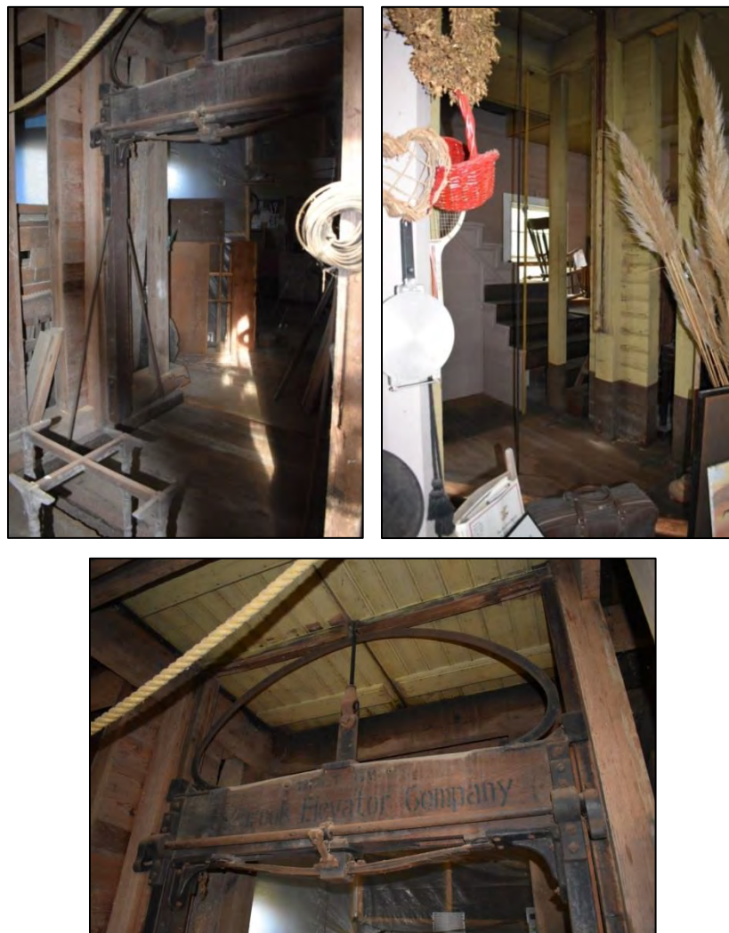
Figure 21: Left, view of elevator sitting on ground floor; to right, view of elevator opening on first floor; center, detail view of “Westbrook Elevator Company” mark.
