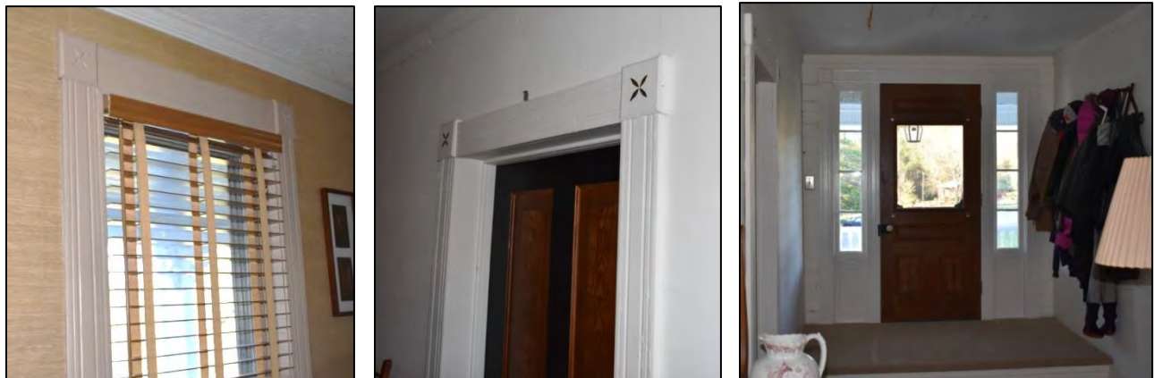
Figure 16: Left and center, detail views of original window and door surrounds found throughout the first and second floors of the house; right, view of original second floor door and sidelights.
