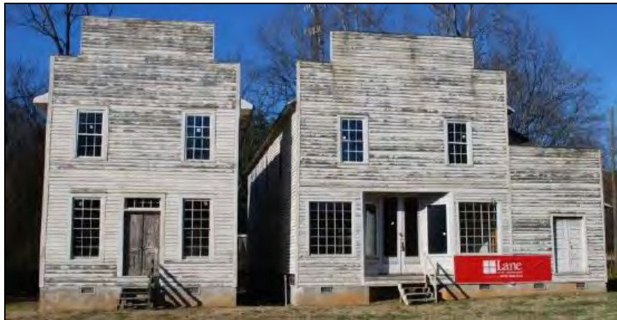
Figure 34: Connelly and McGalliard Stores (BK0385) 6527 Main Circle Street, Connelly Springs, ca. 2012 (photographer: Heather Fearnbach).
