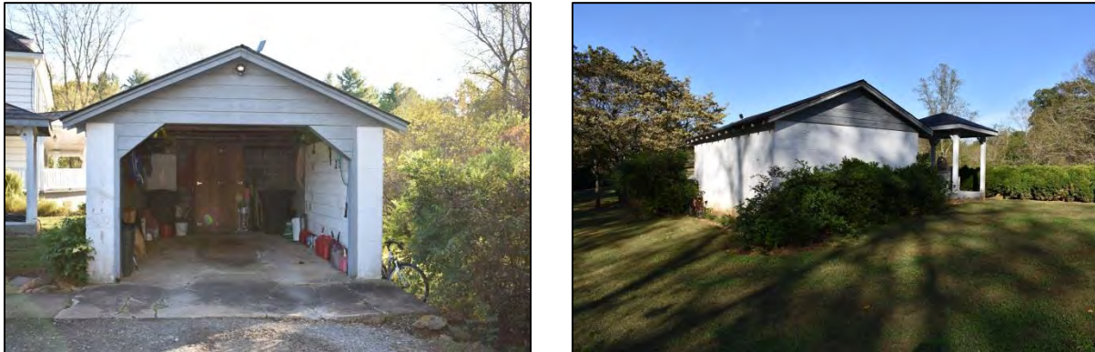
Figure 22: Front (northern) elevation of garage, at left; at right, north rear and west side elevations of garage with well house to right
